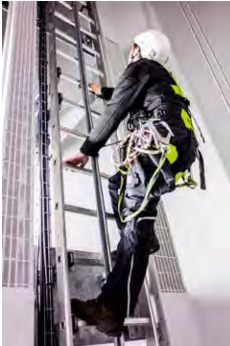
*Figure 1: Ladder and Fall Arrests*
