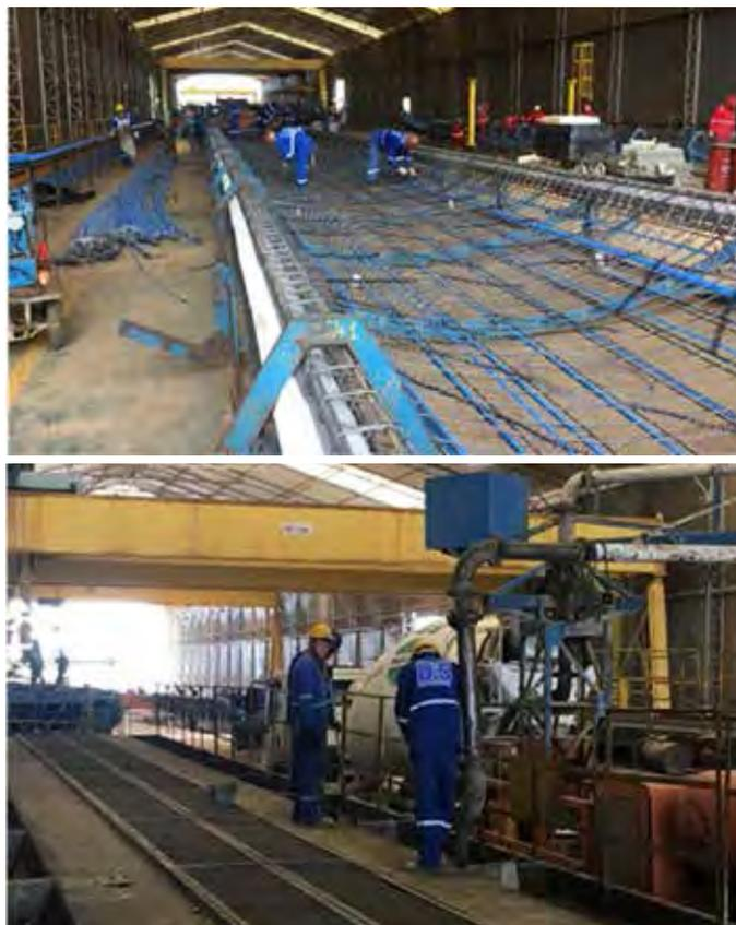
Figure 9 and 10: Reinforcement of the panels. Concreting of the panels
