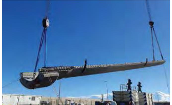
**Figure 19: Tilting of the panels**
