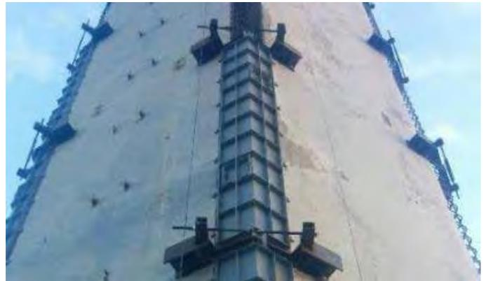
**Figure 20: External jacks on vertical joints**
