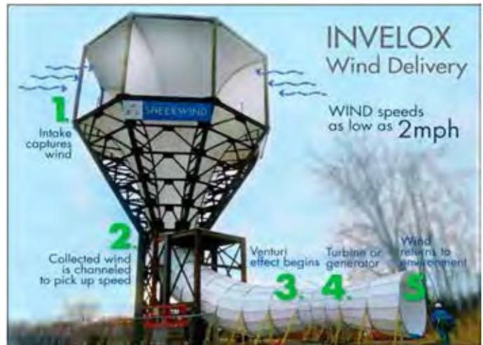
Figure 8: Wind Tunnel Turbine<sup>13</sup>
